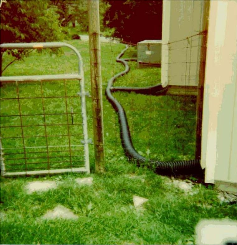
Figure 5. Temporary use of corrugated plastic drainage pipe carry roof water away from foundation wall to several downspout leaders.
