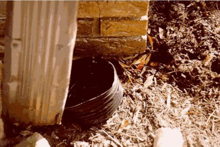
Figure 2. Roof downspout leader pulled away from drain pipe, causing roof water to fall, collect and soak into the foundation soil and weaken the footer's ability to support the foundation wall.
