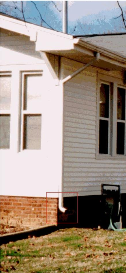
Figure 4. Roof water is improperly directed from roof downspout leader toward foundation wall.
