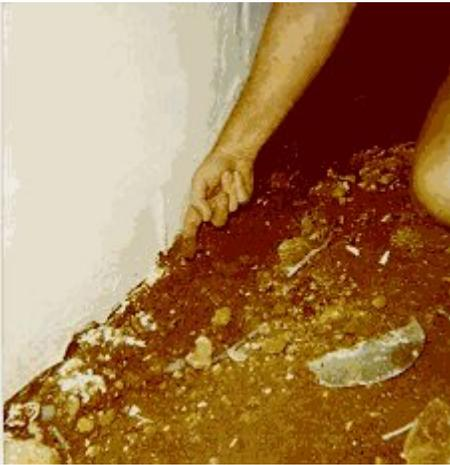
Figure 1. Outside seepage water entering crawlspace area from under foundation wall.
