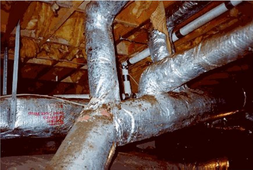
Figure 3. Classic example of mildew formed on heating & A/C ducts (brownish-gray areas) due to high humidity and poor ventilation. Note insulation falling away from underflooring area because of high moisture content.
